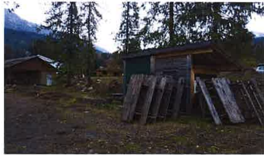
Figure 1 Existing Buildings at Lakeside Campground.
