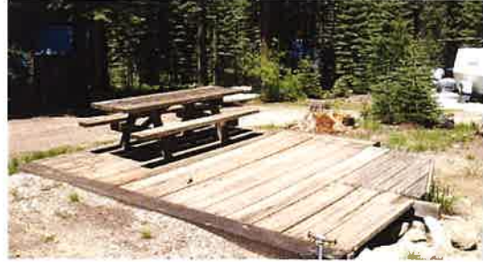
Figure 7 Example of Wood Decking.
