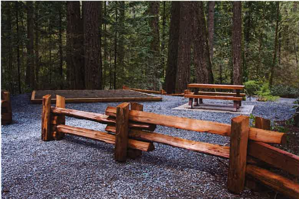
Figure 6 Example of Split Rail Fencing at Campsite from Goldstream Provincial Park.
